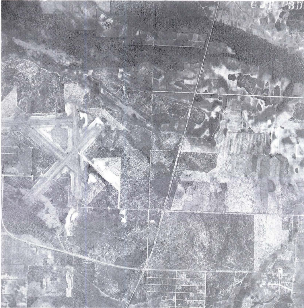
This 1949 view of Prospect Satellite Field, also known as the Fort Lauderdale Executive Airport, shows the airport bounded by Commercial Boulevard on the south and the Seaboard Railway tracks to the east.
