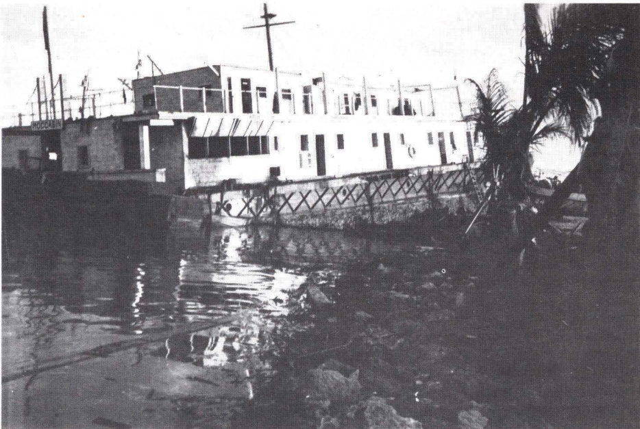
The Coast Guard boat Moccasin served as base headquarters until it was swept across the Intracoastal Waterway and driven ashore at Idlewyld by the September 18, 1926, hurricane.
