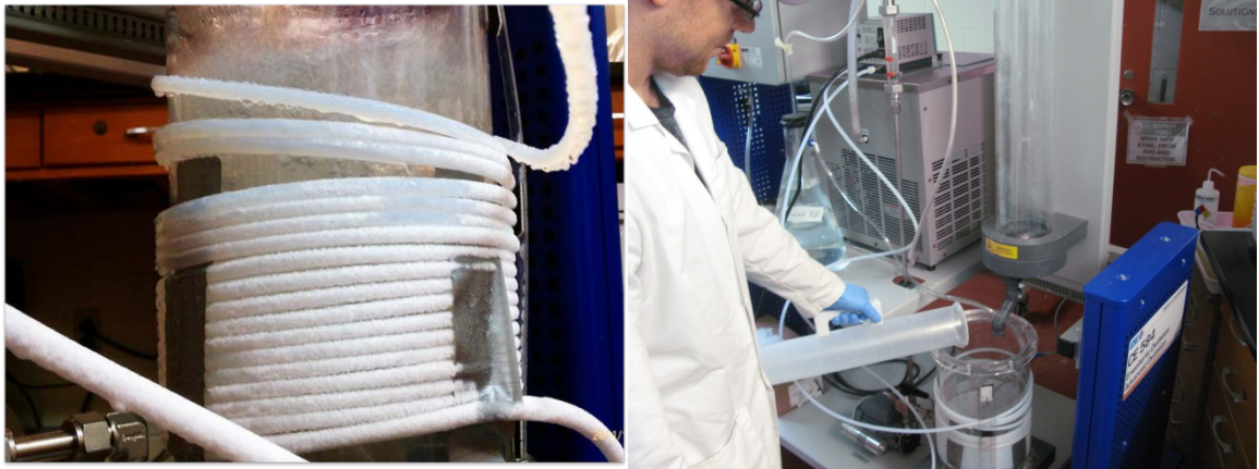
Figure 18: Recirculating cooler hose surrounding leachate reservoir (left) and Frank Youngman testing the temperature control system provided by the recirculating chiller unit
