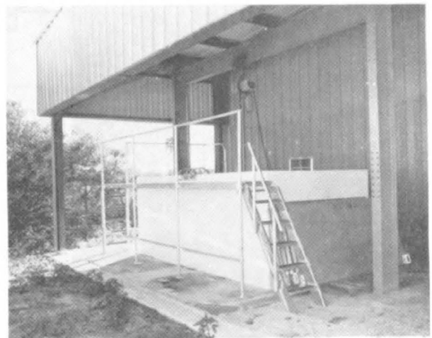
FIGURE 5. CHAMBER CONTAINMENT PIT
