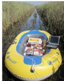
Figure 2. GPR setup in the field showing 250 MHz shielded antenna, ProEx control unit, and laptop
