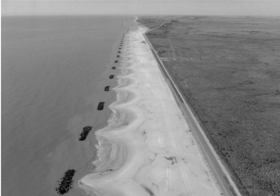
Figure 5. Holly Beach breakwater field, looking west from Louisiana towards Texas. The subaerial beach in this aerial photograph was constructed using sands buried in an offshore channel located about 3.5 miles offshore. Note the prominent salients forming in the lee of the emergent segmented breakwaters.
