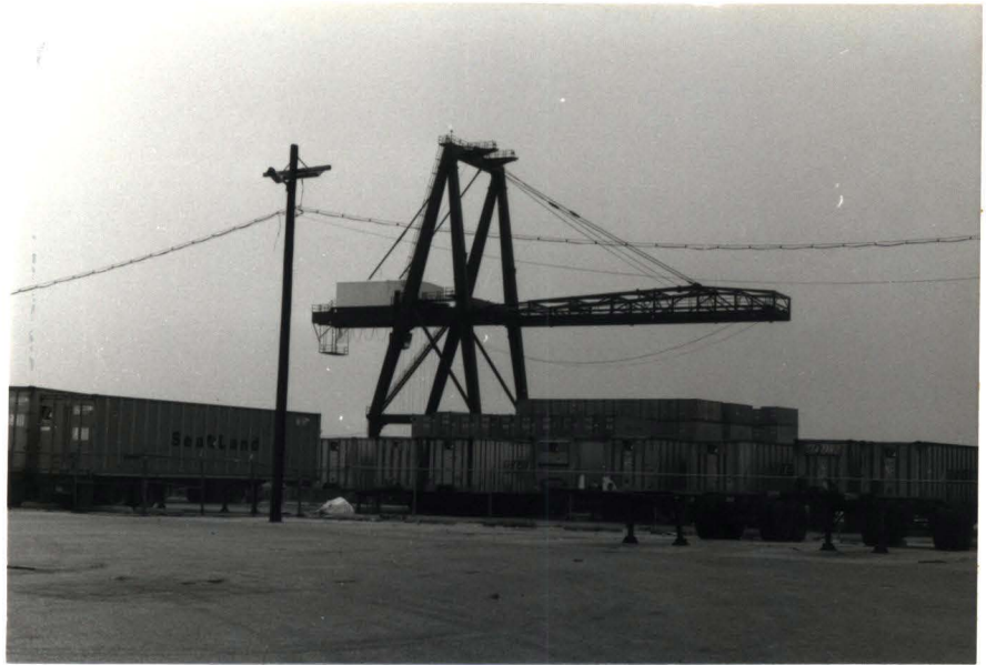
Figure 9. Open storage (containerized cargo).
