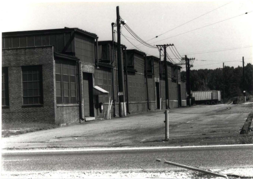
Figure 40. The roof of this warehouse is similar in appearance to a light fabrication building.
