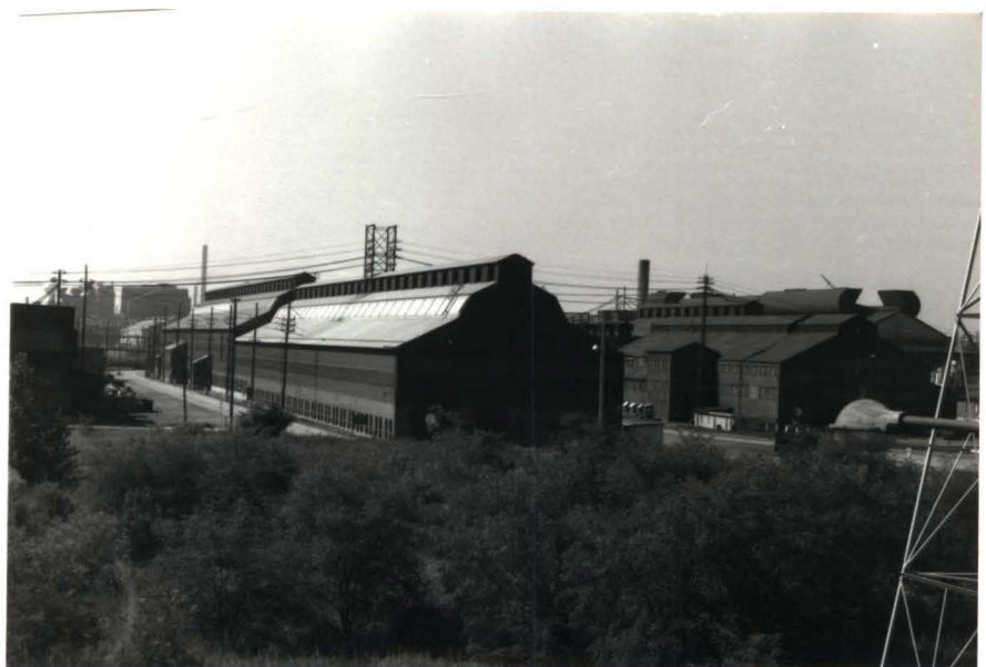
Figure 18. Heavy fabrication (structural steel).
