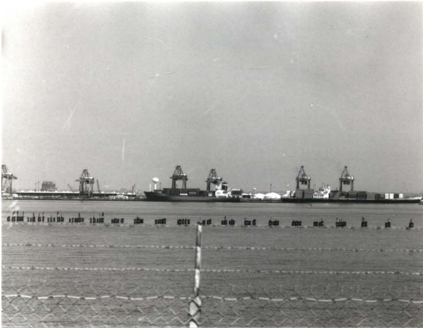
Figure 31. View of the containerized cargo terminal at (B) shown in Figure 30.
