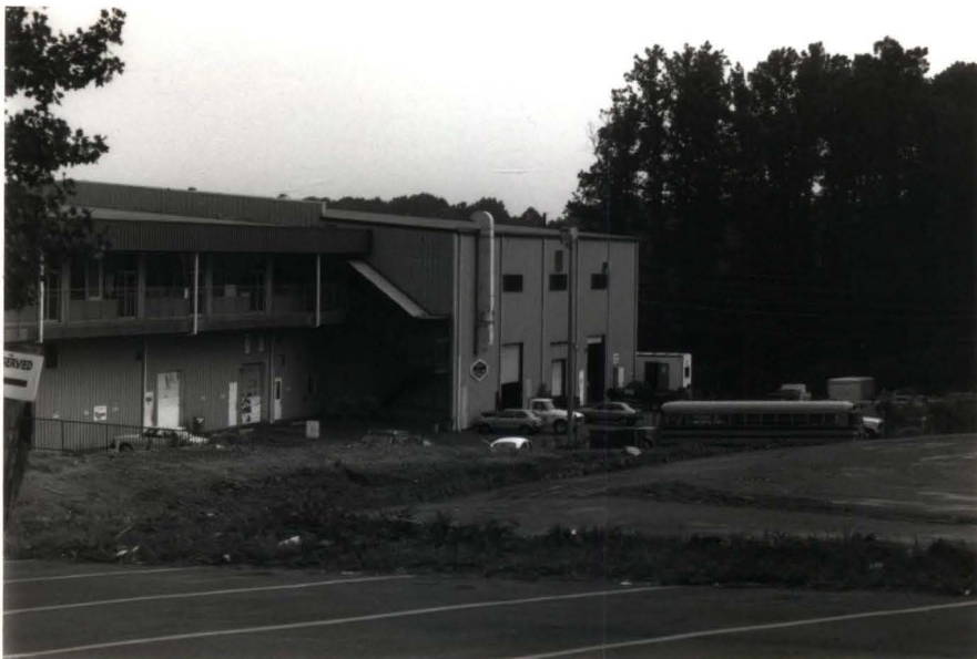
Figure 41. This light fabrication building lacks distinctive features which increases the probability of it being misidentified as a warehouse.
